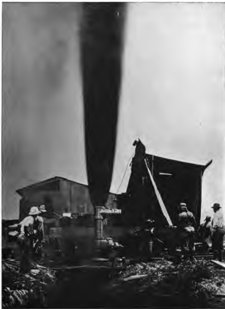
VALVE COMPLETELY OVER WELL.
