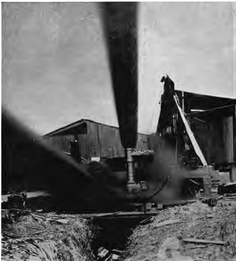
VALVE PARTIALLY OVER WELL.
